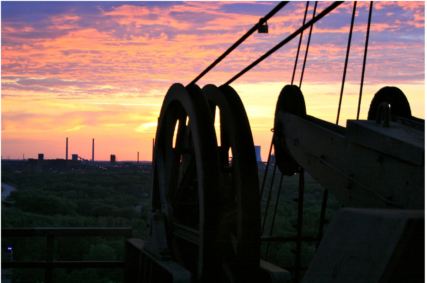
Blast Furnace 5, Landscape Park Duisburg Nord, Germany
